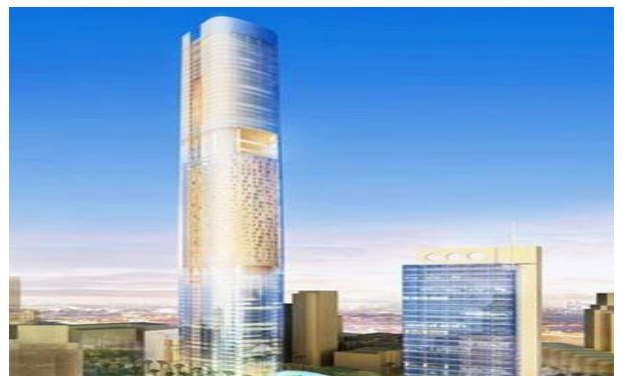
Four Seasons Hotel Tower 2, India PEC cast-in channels
