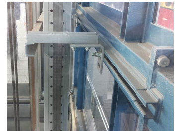
PEC framing channels can be welded directly to the steel components
